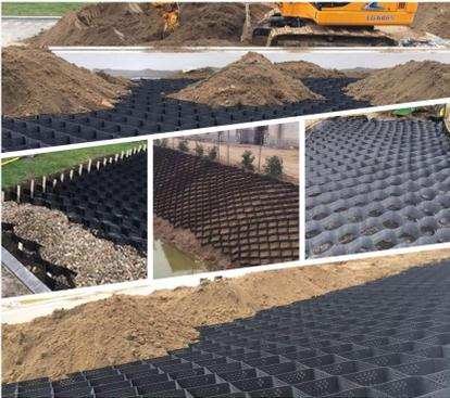
A collage of four photographs showing various applications of the geo grid. The top photo shows a large-scale construction site with a yellow excavator and a large area of the grid being laid out. The bottom-left photo shows the grid used for a drainage ditch. The bottom-right photo shows the grid used for a parking area. The bottom-center photo shows the grid used for a slope stabilization project. |
