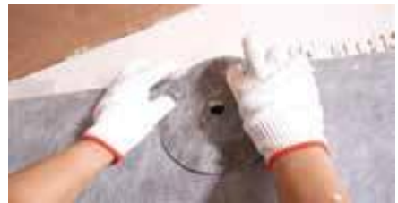
Cover the mixing valve seal
