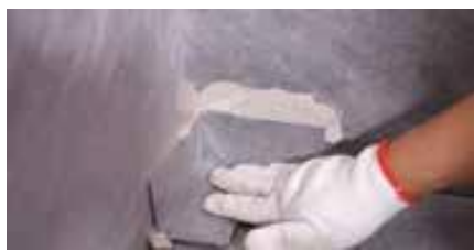
Install the waterproofing corners 1
