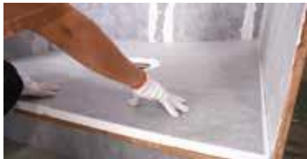
Embed the tray in the mortar
