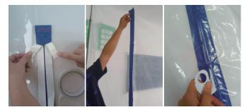
①Flow the "stick this side" sign and stick the double sided tape on the magnetic zipper door.Leave a small gap in the middle of zipper in case the glue stick together.
