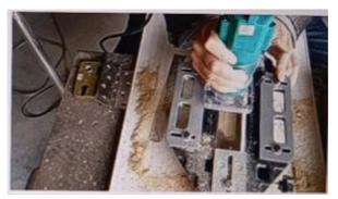
6. There is a certain chance that the edge of the door will be damaged when grooving (The material of the wood and the work of the cutter head may cause it), so don't hollow out all the wood at the edge.
