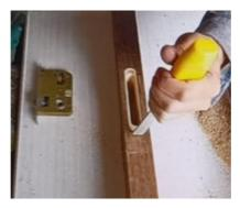
5. Complete the slot and install the lock body guide plate.
