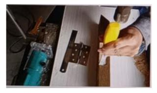
8. Finish slotting and install the hinge.
