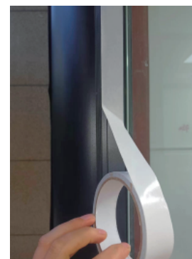
2. Peel off the release paper
