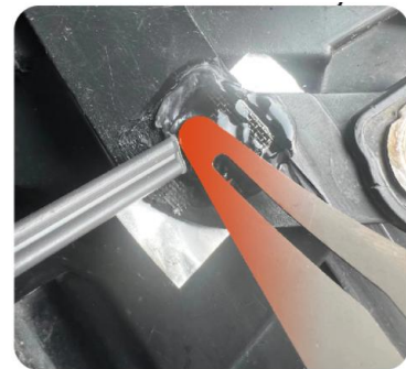
5. Melt welding rod to cover the whole repair net
