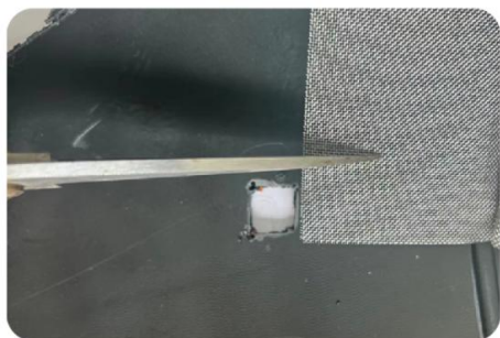
1. Cut stainless steel repair net
