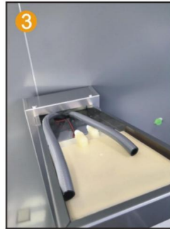
3 Connect PVC pipes and LED light wires through the hole
