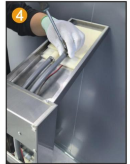
4 Fix the PVC pipe with a throat clamp on the top spray joint
