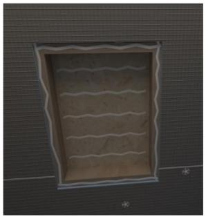
4. Seal joints between Niche and backer board with waterproof Sealant.
