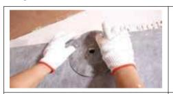
Cover the mixing valve seal(Not provide)
