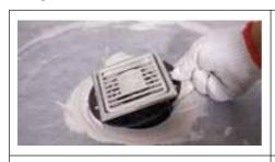
Install the drain adjustment ring(Not provide)
