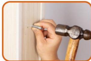
8. Insert the expansion glues to all holes.
