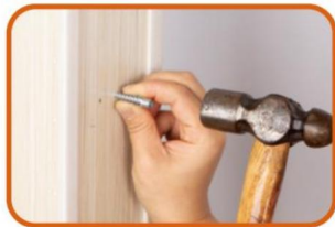
8. Insert the expansion glues to all holes.
