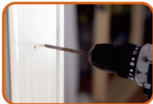
7. Drill holes of with an electric drill as the marks.
