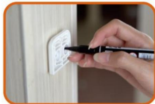
6. Mark the holes position of the two brackets and then pull out the two brackets from wall.
