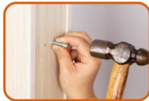
8. Insert the expansion glues to all holes.
