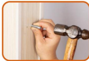
8. Insert the expansion glues to all holes.
