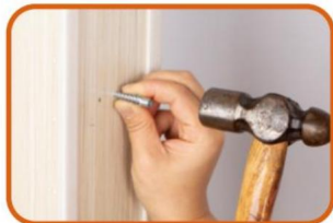
8. Insert the expansion glues to all holes.
