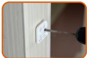
9. Drill the two Brackets to wall as the holes.
