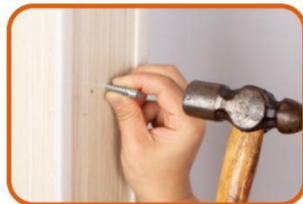
8. Insert the expansion glues to all holes.
