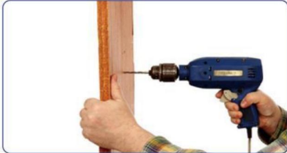
1. Drill bolt holes in fixed piles with electric drill
