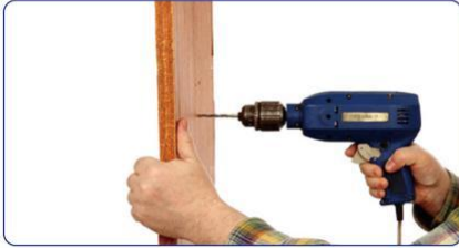
1. Drill bolt holes in fixed piles with electric drill
