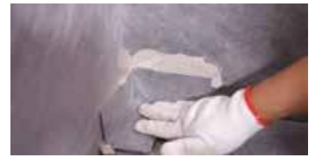
Install the waterproofing corners 1
