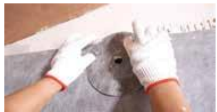
Cover the mixing valve seal
