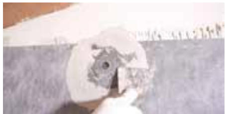
Make the surface even
