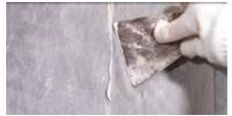
Make the wall surface even
