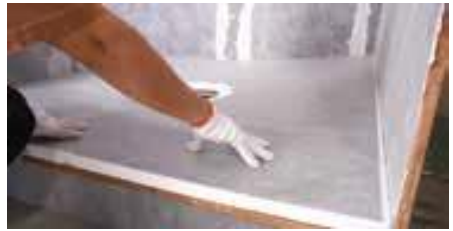
Embed the tray in the mortar
